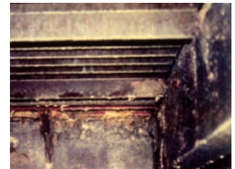
Corrosion caused by microorganisms
